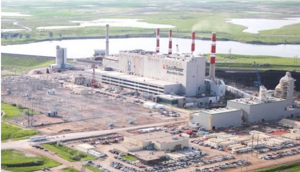
CCS plant, Boundary Dam, Canada
